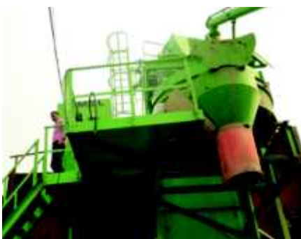
NHAI construction site and the RMC plant
